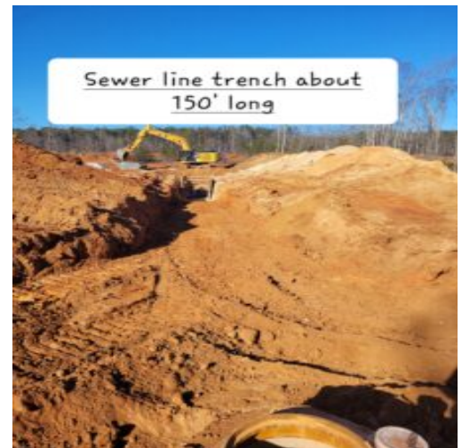
Deep trench dug for sewer line
