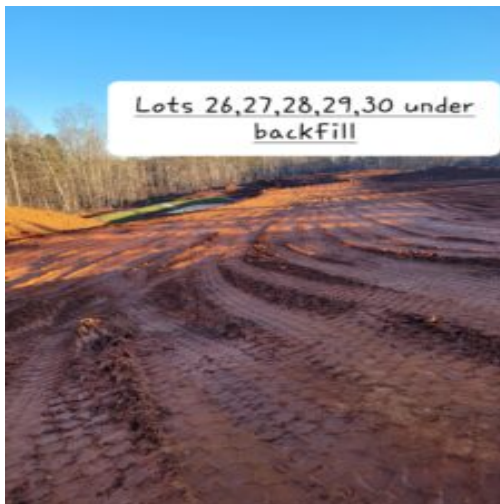
Picture showing building pads under backfill stage
