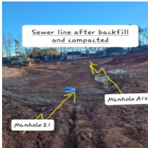
Sewer line between Manhole A12 and E1 after backfill
