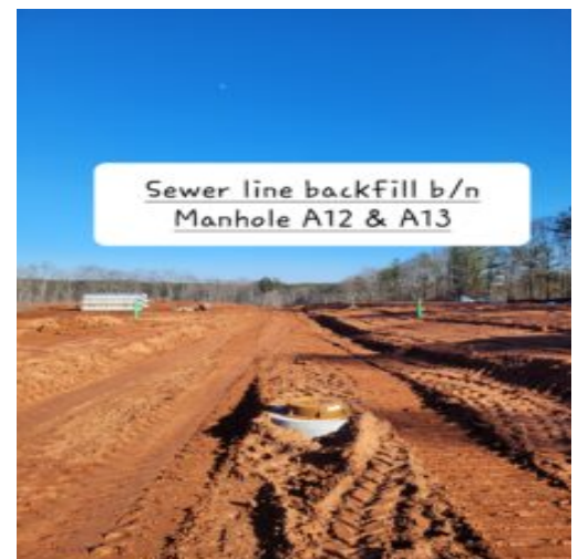
Sewer line backfilled and compacted
