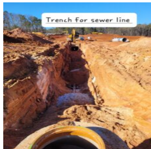
A deepn trench for sewer line between manholes A12 and A13
