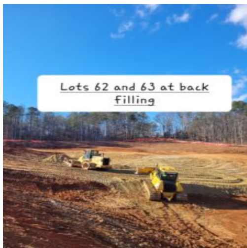
Picture showing lat 62 and 63 under backfill and compaction.
