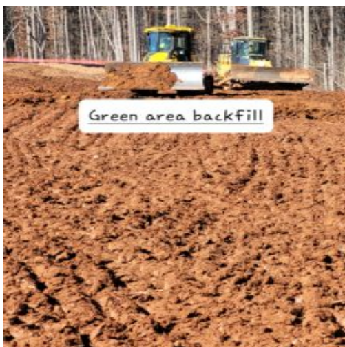
Picture showing green area backfill
