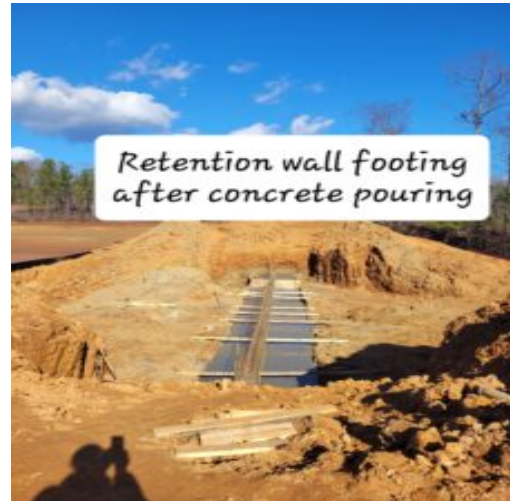
Picture showing a 76x8 feet retention wall footing
