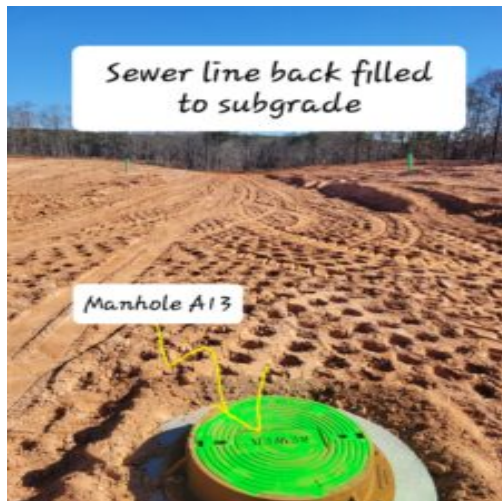
Photo depicting from Manhole A13 towards A12
