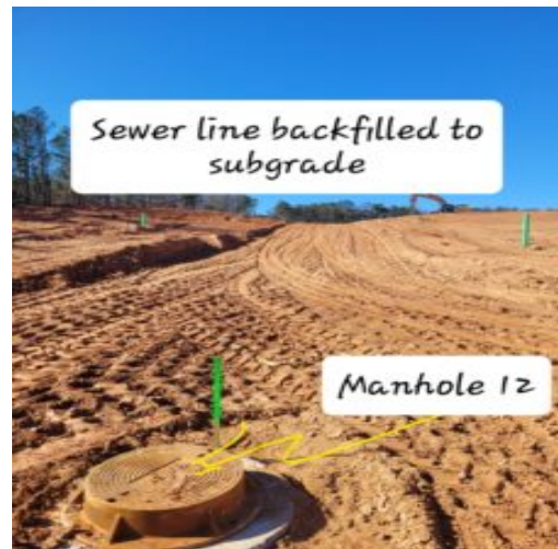
Photo depicting from Manhole A12 towards A13
