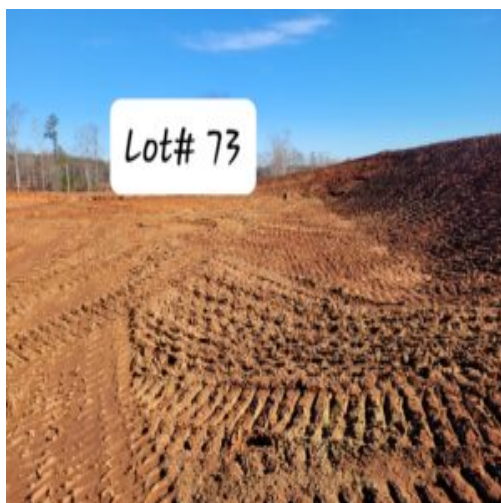
Picture showing lot 73 at subgrade
