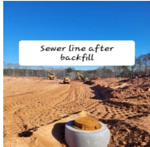
The sewer line after backfilled and packed
