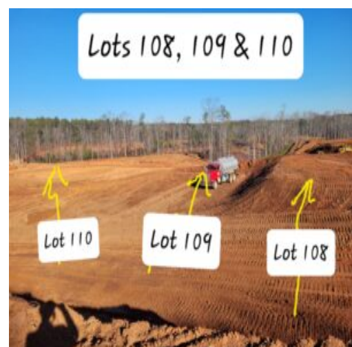
Picture depicting lots at subgrade
