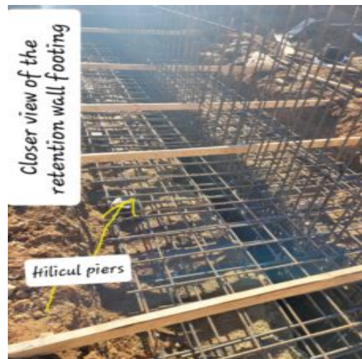
A closer view of the footing to show the Reenforcing hilicul piers
