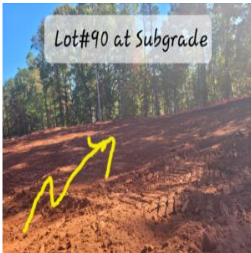
Lot 90 is well done to subgrade
