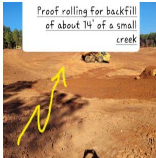
The fill at the small creek started after doing proof rolling
