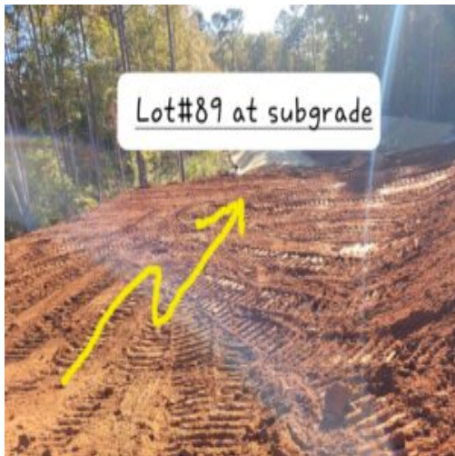
Lot 89 is also done to subgrade
