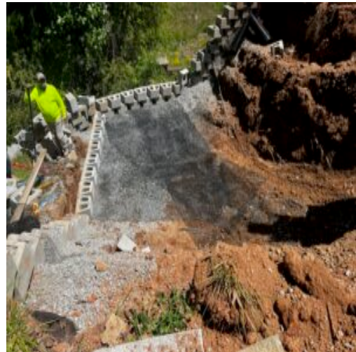
Installation of Geosynthetic reinforcement
