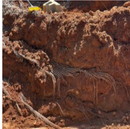
Removal of Geosynthetic reinforcement
