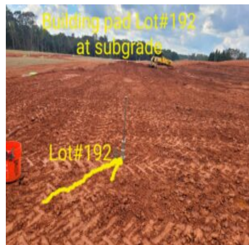
One of the bldg pad were drive cylinder test is taken
