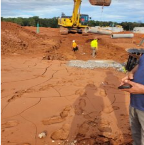
Storm line back fill b/n manholes B13 and B13.1
