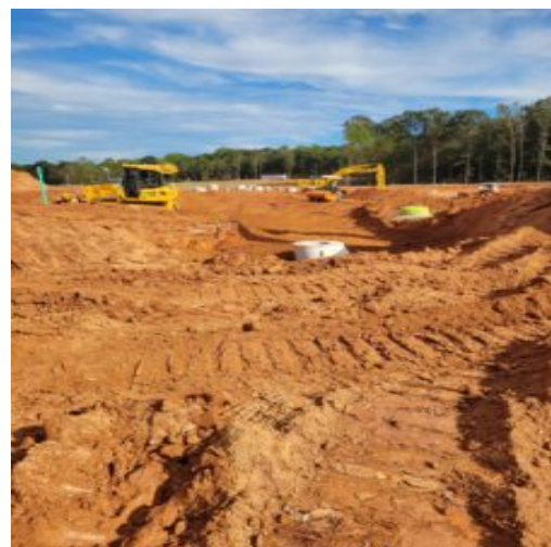
Sewer line back fill between F2 and F1 manholes
