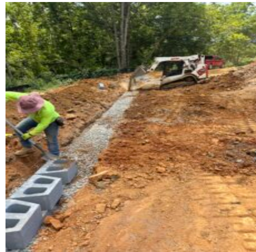
First course placement
