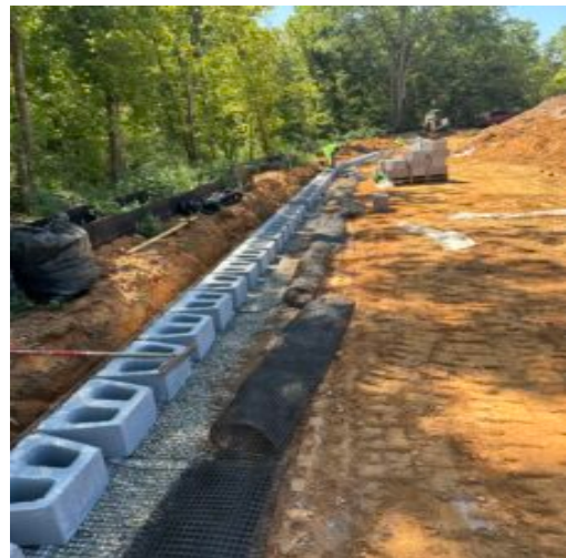
Wall looking South
