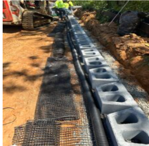
Matting and drain placement
