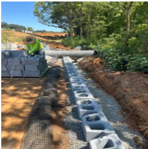
wall looking North
