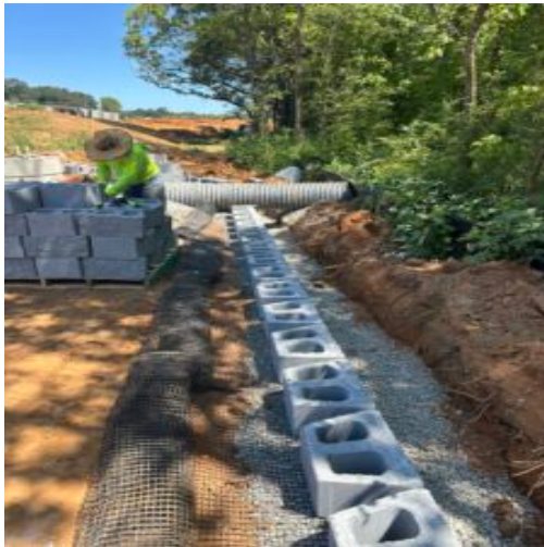
wall looking North
