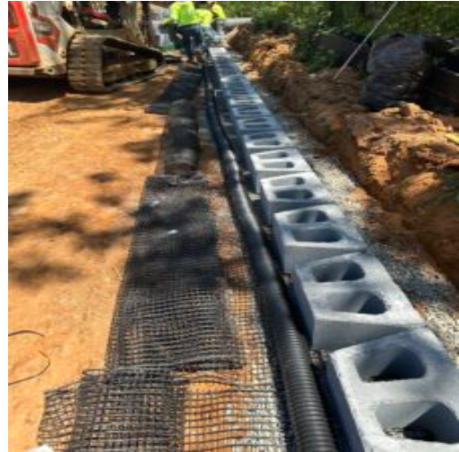
Matting and drain placement
