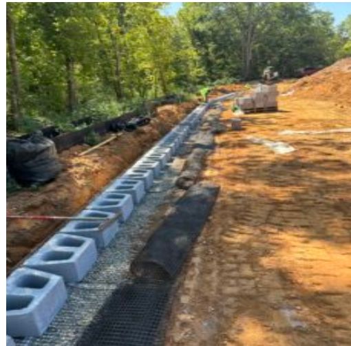
Wall looking South
