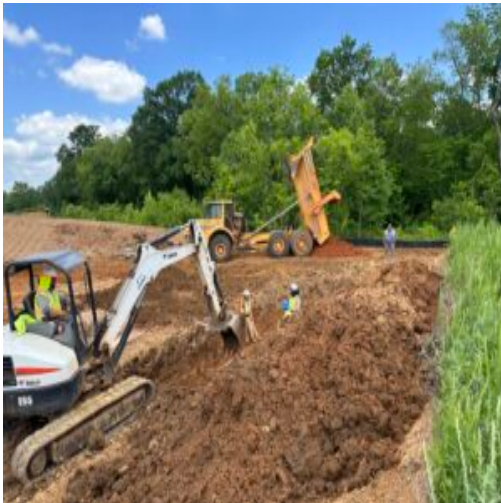
Burrito wrap excavation/ replacement with dry soil
