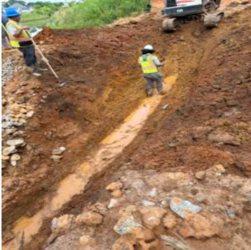
burrito wrap excavation
