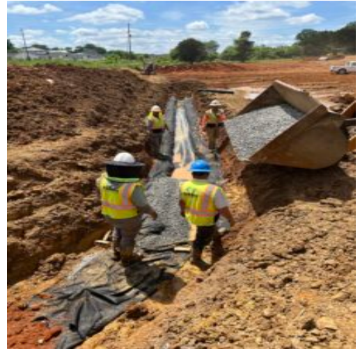
Installation of 57 stone in burrito wrap
