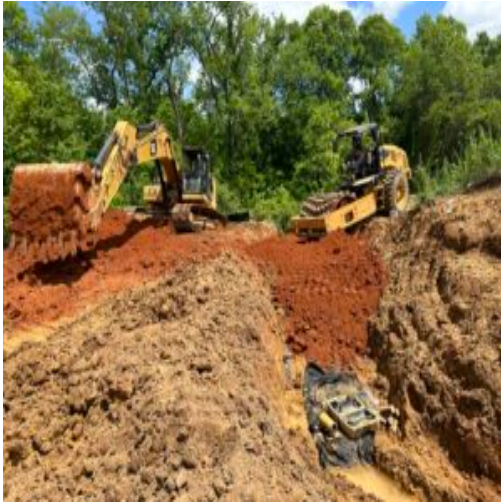
Back filling for temporary road at burrito wrap
