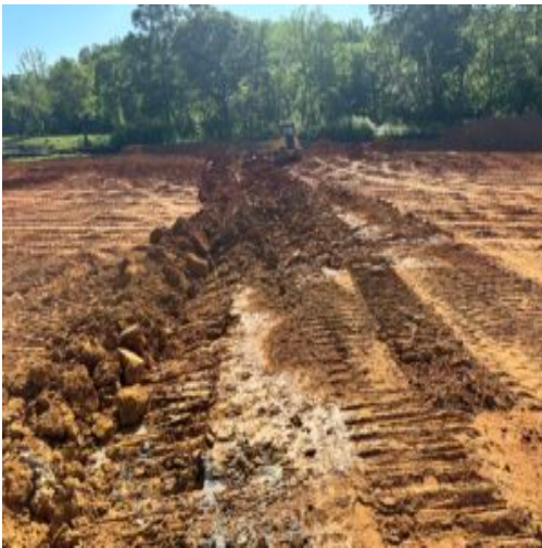
area 1 being scarified
