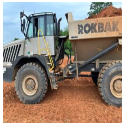
proof roll with loaded off road dump truck
