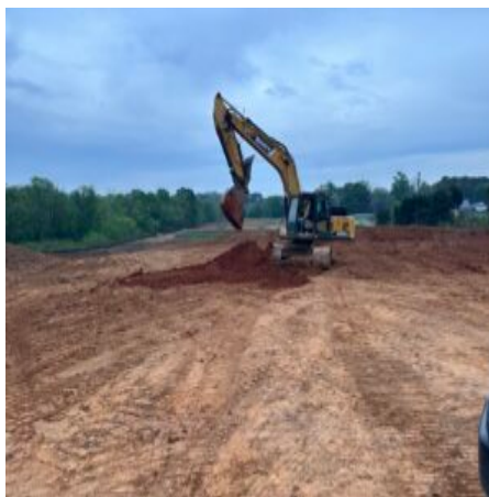
excavating for proctor
