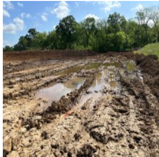
future area of Lots 54-61 plus roadway and sidewalk with uncontrolled ground water
