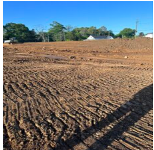
Lots 95,95,97 underground water
