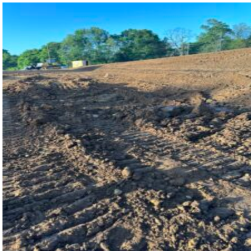
lots 95,96,97 underground water
