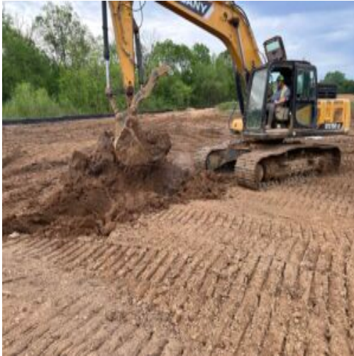
excavating test pits
