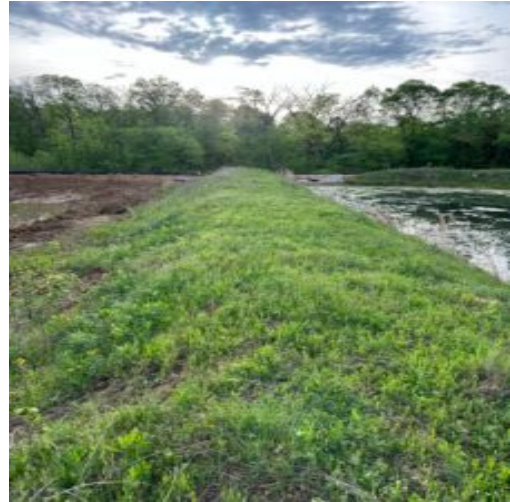
detention pond earth wall
