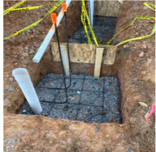
Location of 1st DCP. Rebar and 57 stone was removed.
