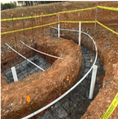
Location of 2nd DCP in curved area (57 stone removed)
