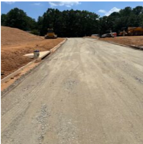
Placed Graded Aggregate Base (GAB)
