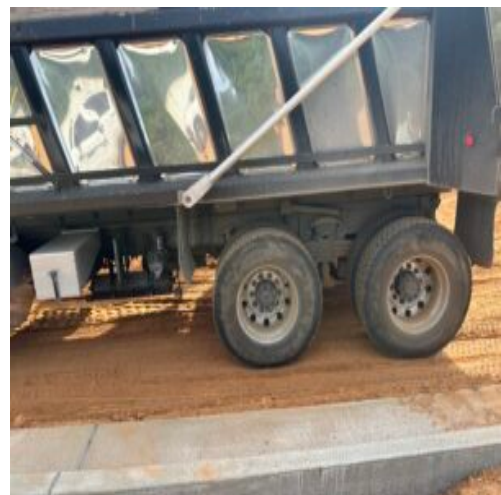
Loaded tandem dump truck proof roll
