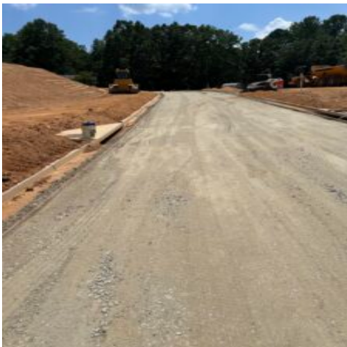
Placed Graded Aggregate Base (GAB)
