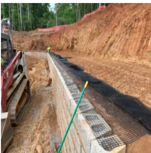
Retaining wall at end of day
