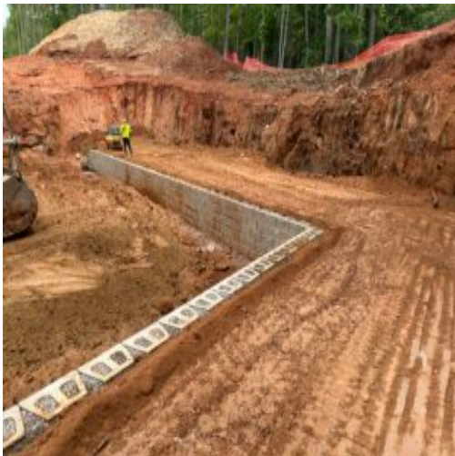
Using trench packer against wall
