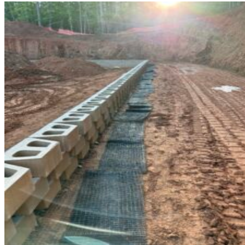
Retaining wall beginning of day with high moisture content on previous days lift.
