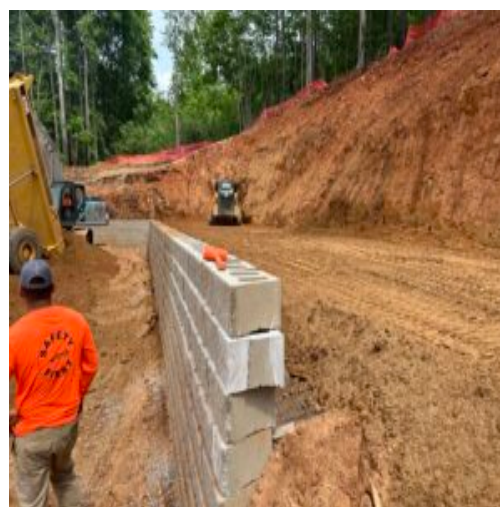
Spreading backfill
