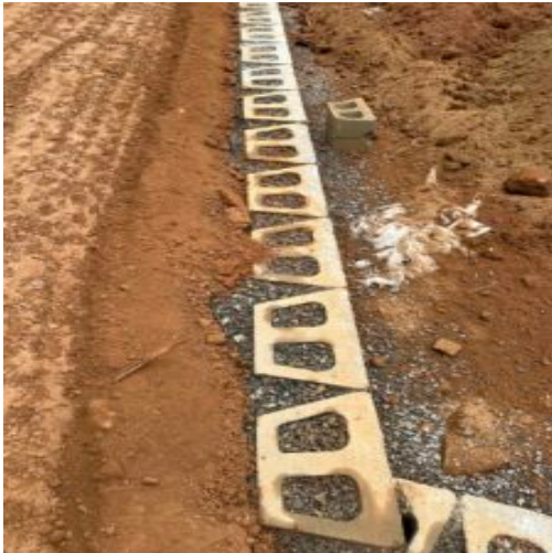
Block filled with 57 stone
