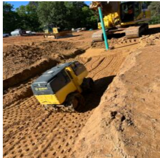
Lot #1 sanitation sewer lateral
