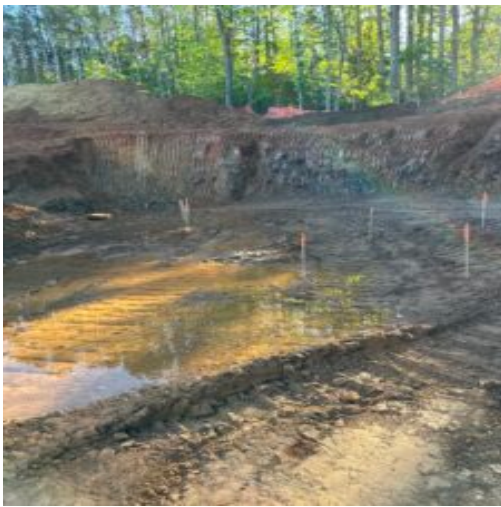
Retaining wall footing on lot #25
