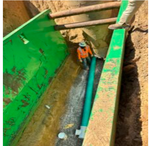
Sanitation sewer placement
