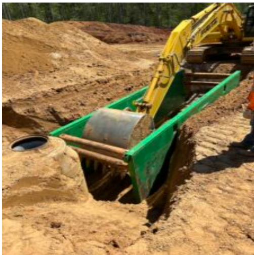
excavation with trench box for sanitation sewer
