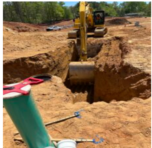
excavation for sanitation sewer
