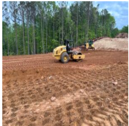
compaction of lots 9, 10 and 11
