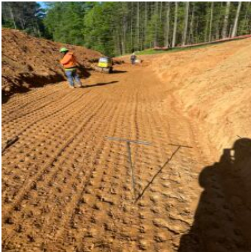
trench packer utilization
