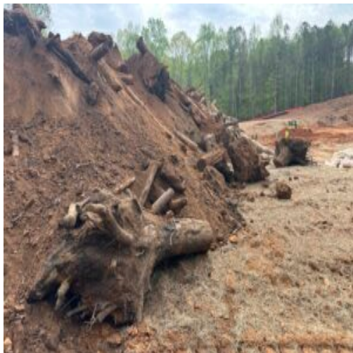
burry pit debris after removal side view
