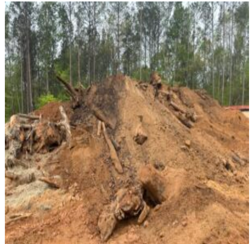
Burry pit debris after removal front view
