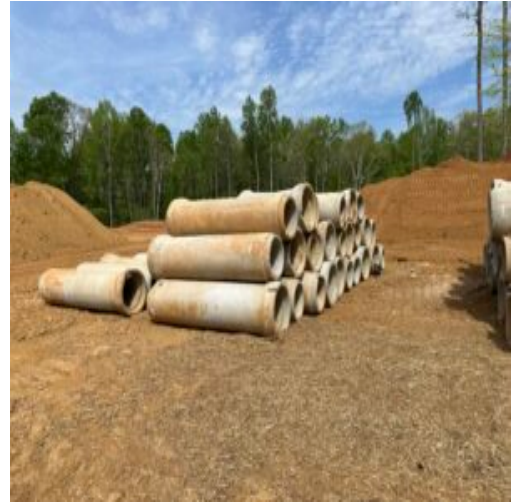
RCP delivered from another job
