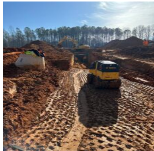
compacting with trench packer
