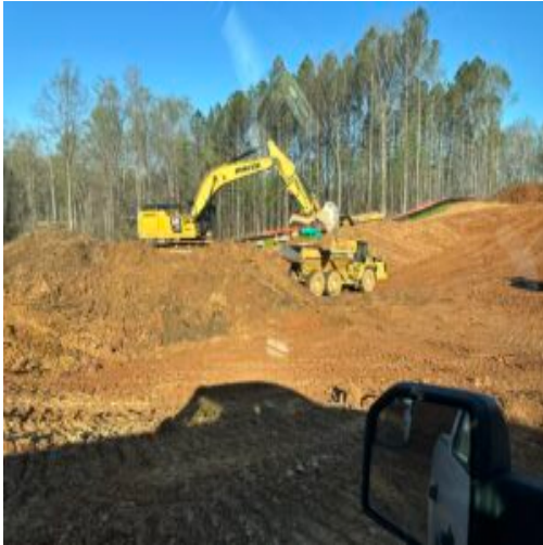
Hauling off topsoil
