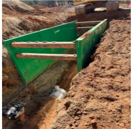
trench box for storm drain placement
