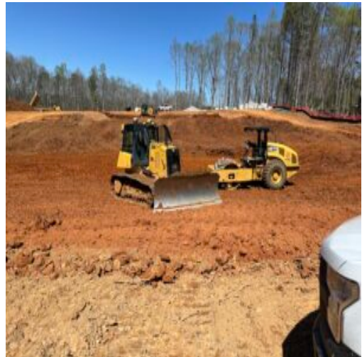
Dozer and compactor
