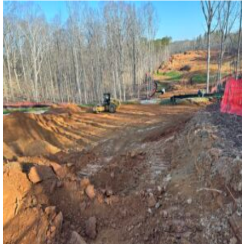
future roadway center of project and testing location
