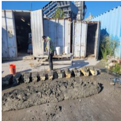
One set of 11 beams
