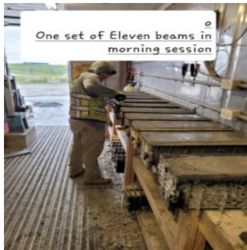
One set of 11 beams
