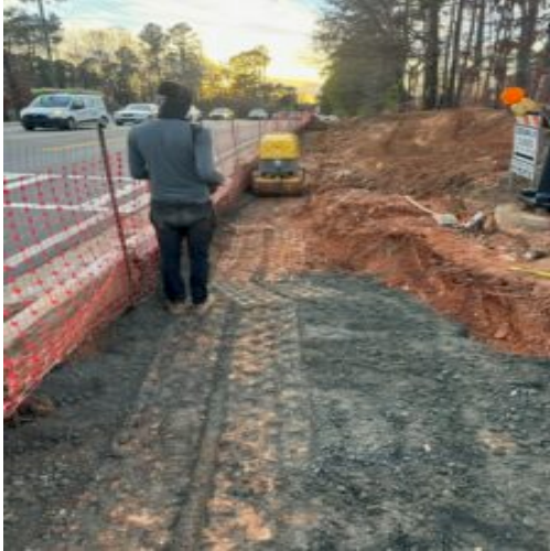
GAB Installation in Acceleration and Deceleration lane
