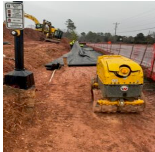
GAB Installation in Acceleration and Deceleration lane
