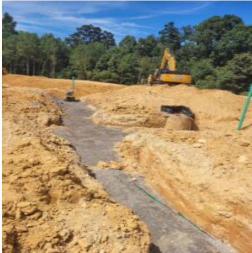
Sewer line filled with gav (rock).
