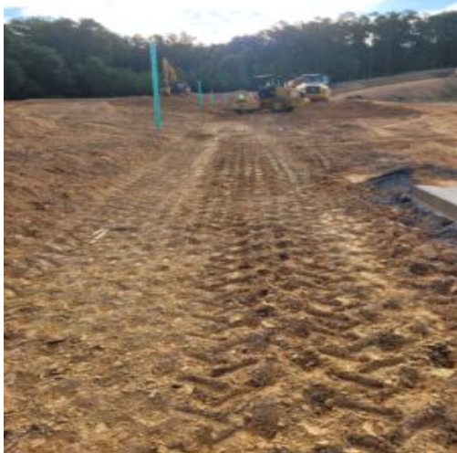
Sewer line backfilled with soil and compacted
