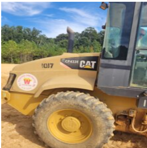
The machine and the model doing soil compaction
