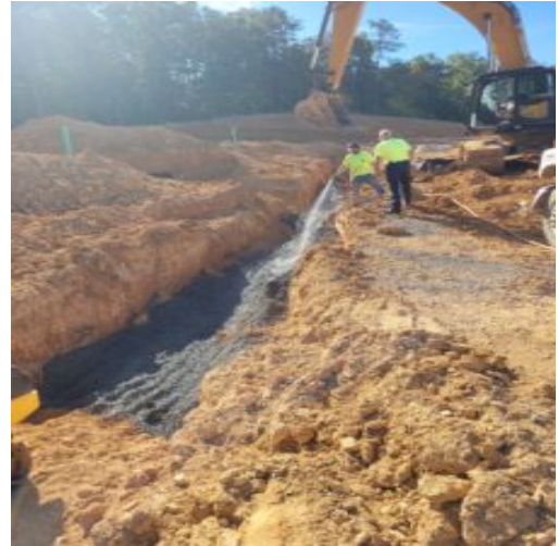
Adding water on gav before compaction
