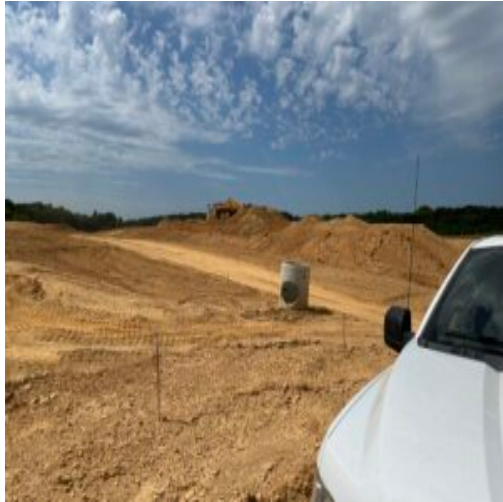
Moving soil stockpile
