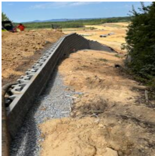
Retaining wall NOT inspected by ASEC
