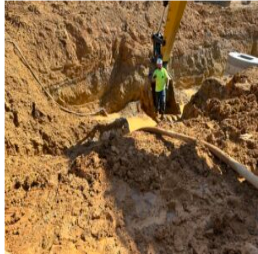
removing corrugated pipe at AI4
