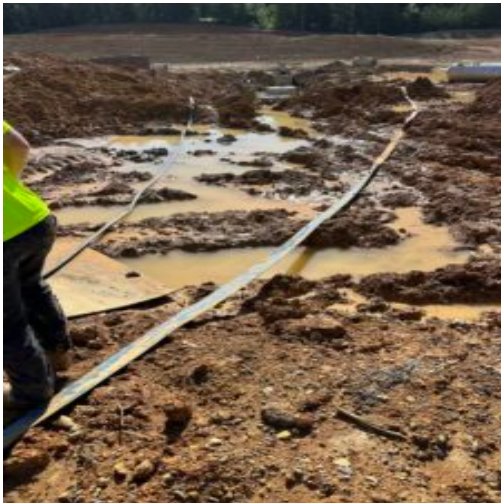
Pump water out of trench
