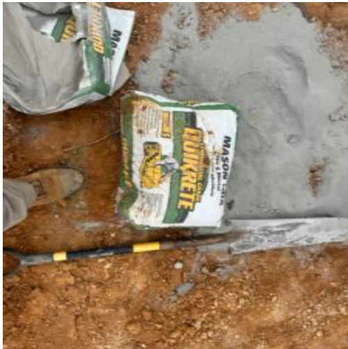
used to seal manholes
