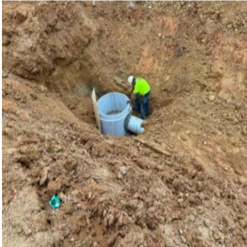
Sealing Manhole
