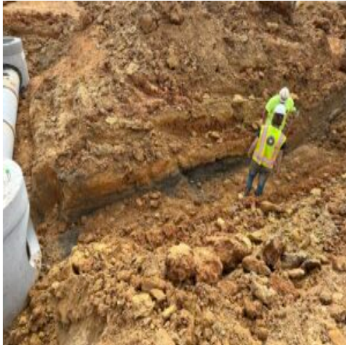
AH2-AHAH# Topsoil covered
