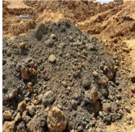
Topsoil removed AH2-AH3
