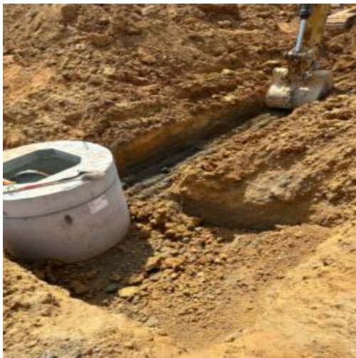
AH3 topsoil exposed
