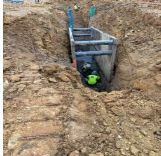
Sanitation pipe placement in trench box (Ductile iron pipe)
