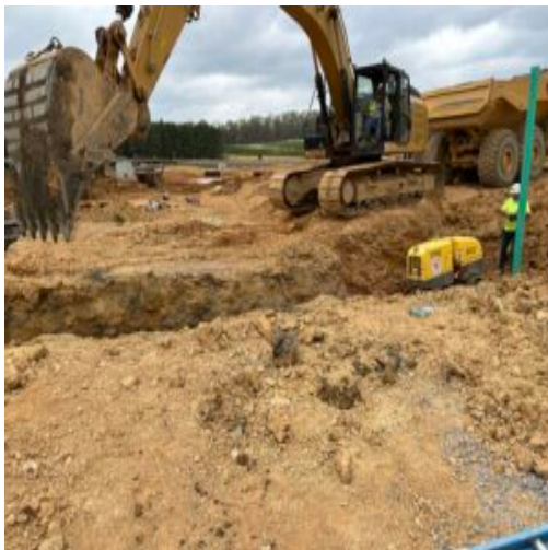
using Trench packer between AH5-AH6 on approximately 4 foot lift
