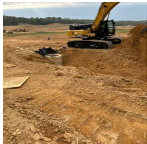
AH5 with approximate 4 foot lift
