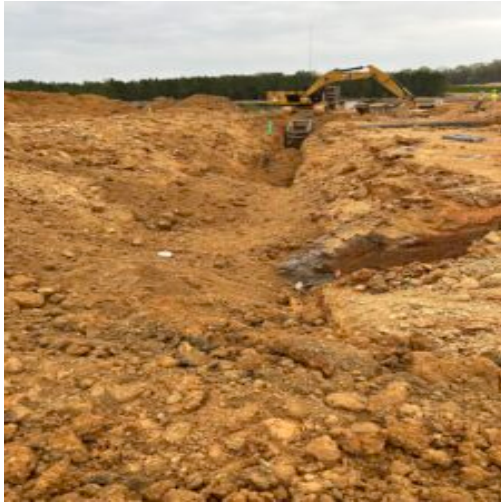
Sanitation pipe with approximately 4-5 foot lifts
