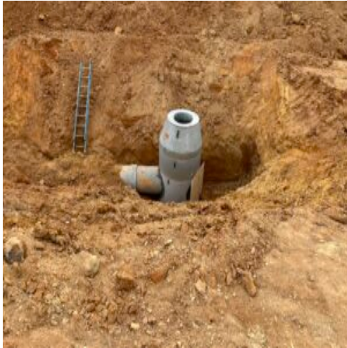
AH6 storm drain manhole
