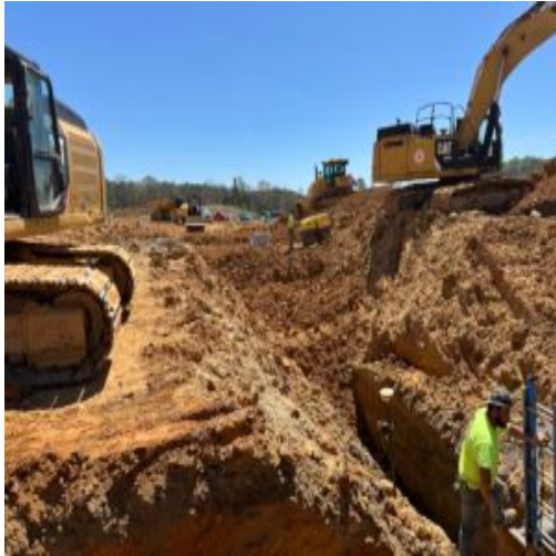
sanitation sewer facing 4.4
