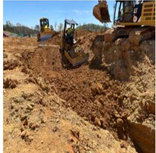
compacting sanitation sewer at 4.4
