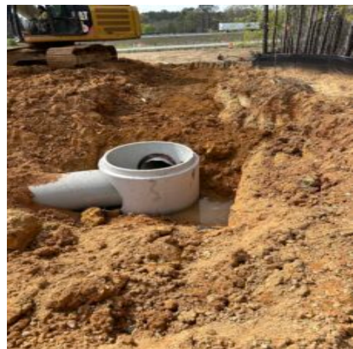
E2 storm drain manhole
