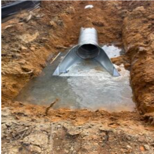
termination of storm drain to roadway
