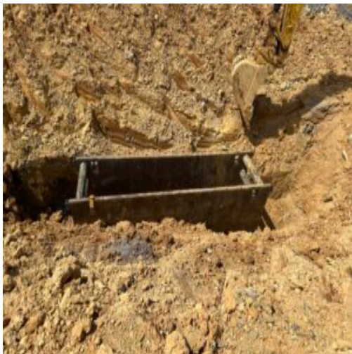
4.3 to 4.4 sanitation sewer
