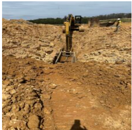
4.3 to 4.4 sanitation sewer
