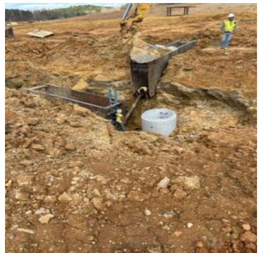
Trench box for sanitation sewer
