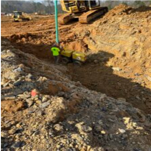
Sanitation lateral sewer placement
