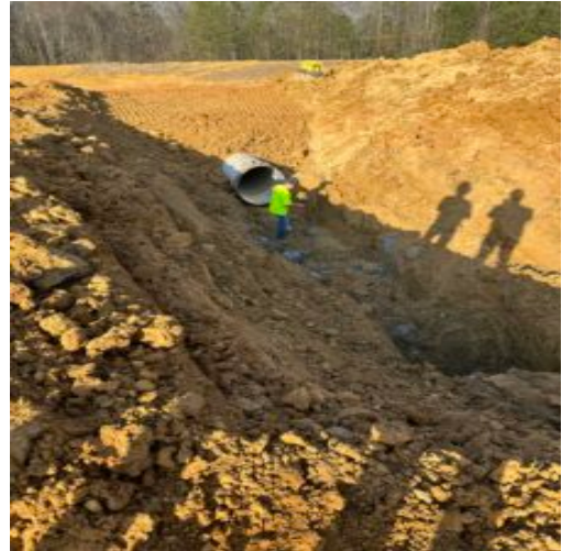
storm drain placement
