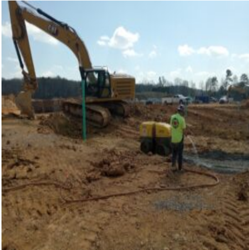
Area 1 adding water to GAB
