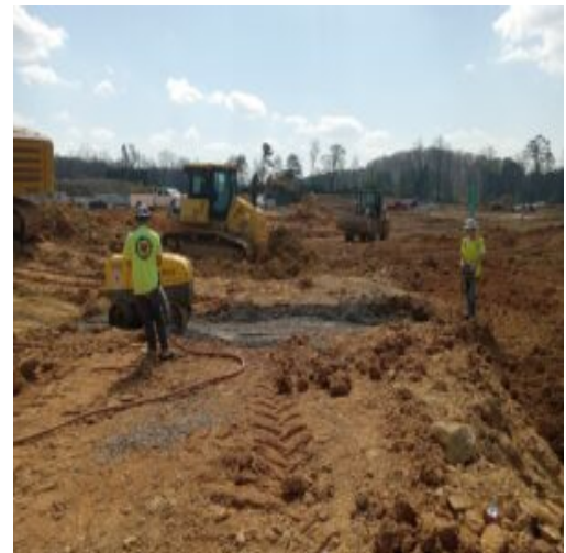
Area 1 Lateral Sanitation Pipe
