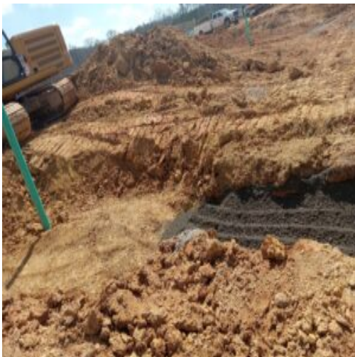
Area 1 Lateral Sanitation Pipe
