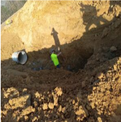
Area 2 before 20 ft of storm drain pipe was installed
