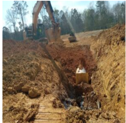
Area 2 after 20 ft of storm drain pipe was installed
