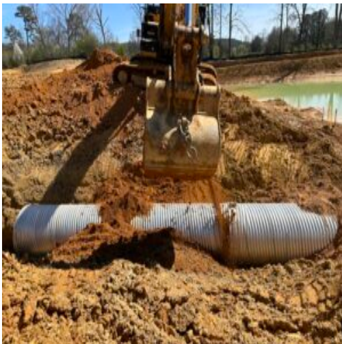
4 feet of fill being placed next to BA1 headwall
