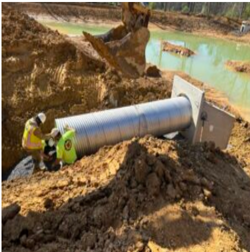
BA1 Headwall and 20 feet of 48 inch corrugated pipe.
