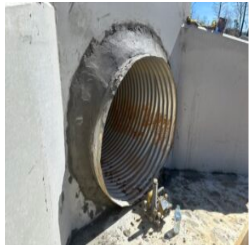
BA1 sealed around pipe
