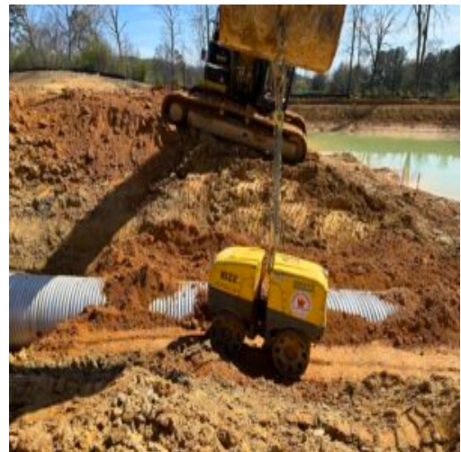
4 feet of fill being compacted with a trench packer.
