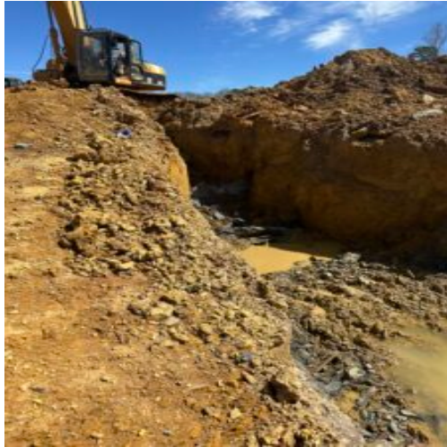
BA1 headwall and storm pipe location
