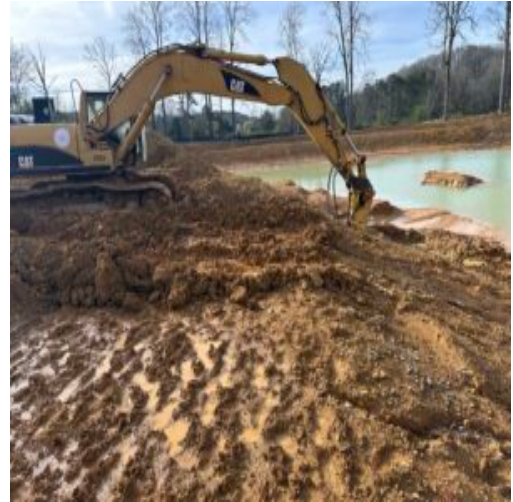
BA1 headwall location
