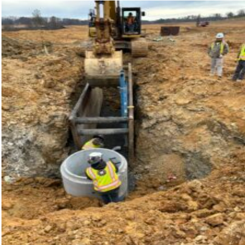
trench box at 1.4
