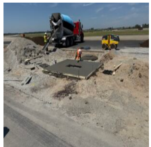
Placed concrete Collar area 1
