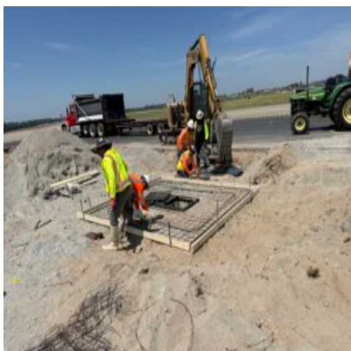
form/rebar collar area 1 observed by 2MNext and AtlNext before concrete placement.
