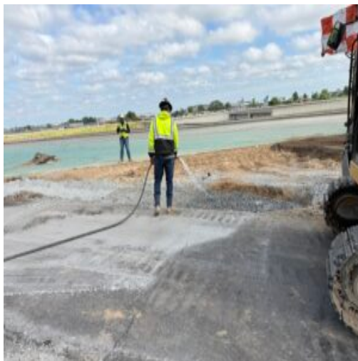
Adding water to GAB
