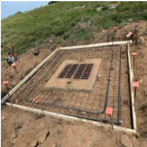
Formed/rebar Collar next to flume observed by 2MNext and AtlNext before concrete placement.
